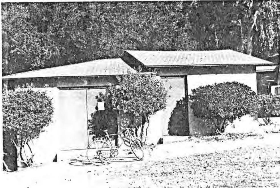
#15a - Storage Building
