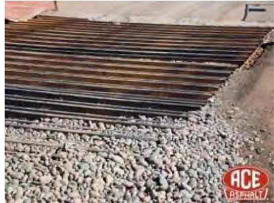
This BMP consists of stabilizing the defined entrance/exit point of the facility to reduce the sediment (mulch and dirt) onto public roads by vehicles. Stabilized entrances/exits are an effective method for reducing the tracking of sediment from the site.
