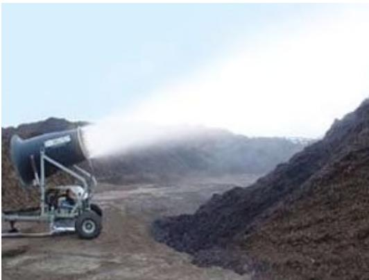
This BMP consists of applying water or other dust palliatives to prevent or alleviate dust nuisance.
