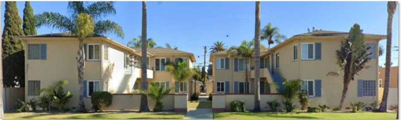
Figure 1 – View of property in 2023 following window alteration (looking east)
