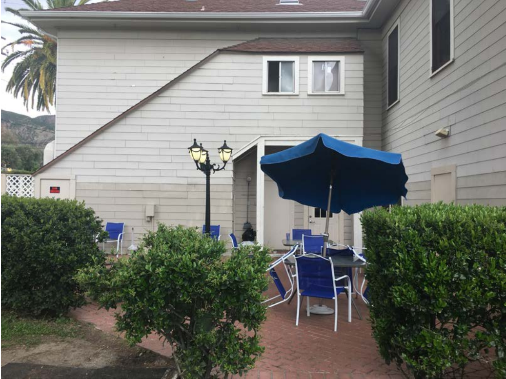
View of Patio (Facing North)
