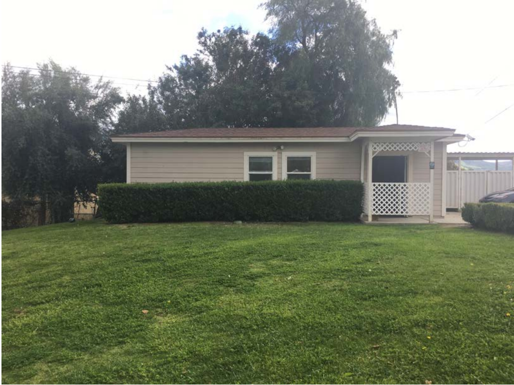
Front of Laundry Structure
