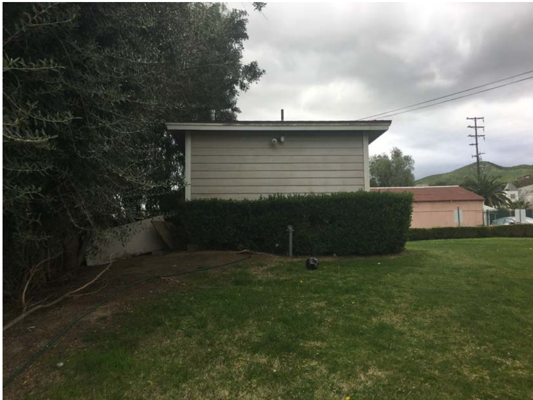
Side of Laundry Structure
