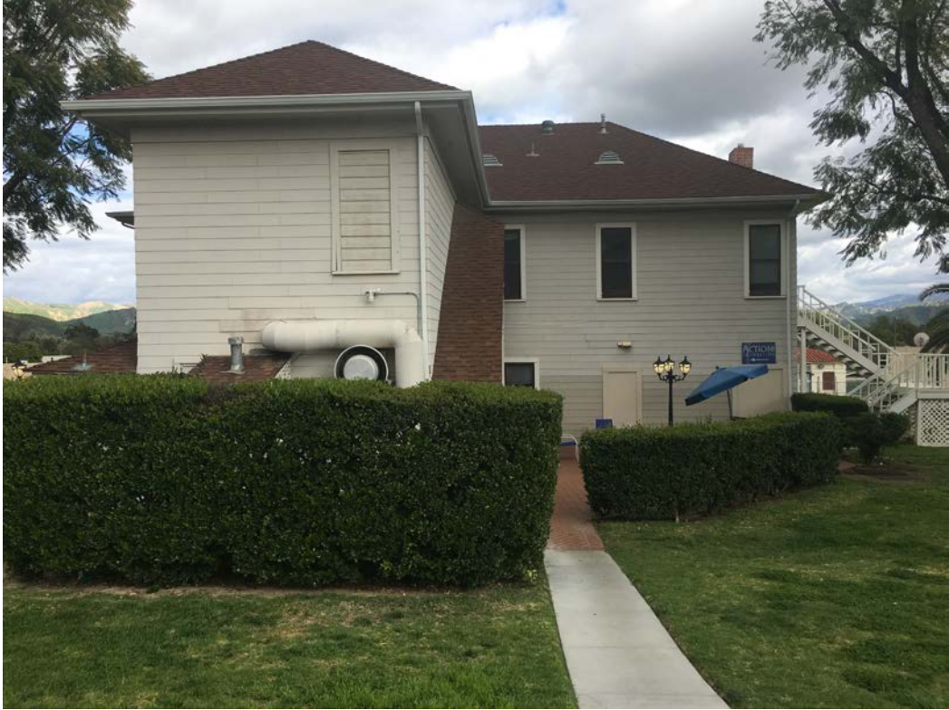
West Side of Primary Structure
