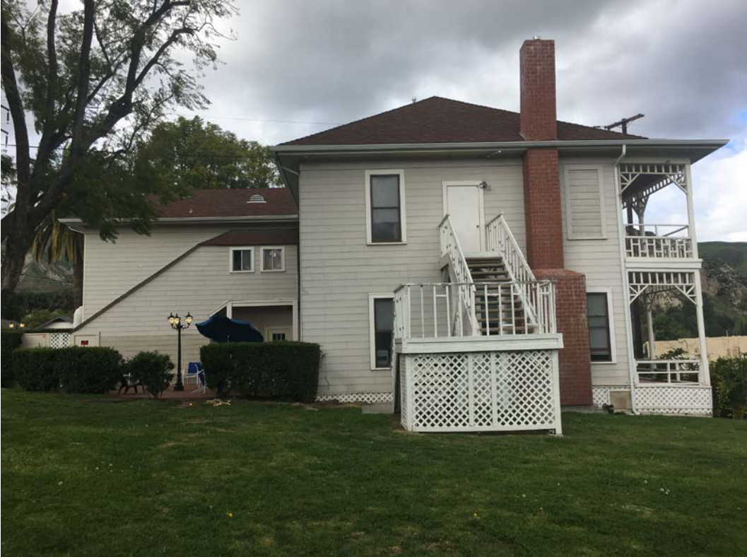
South Side of Primary Structure
