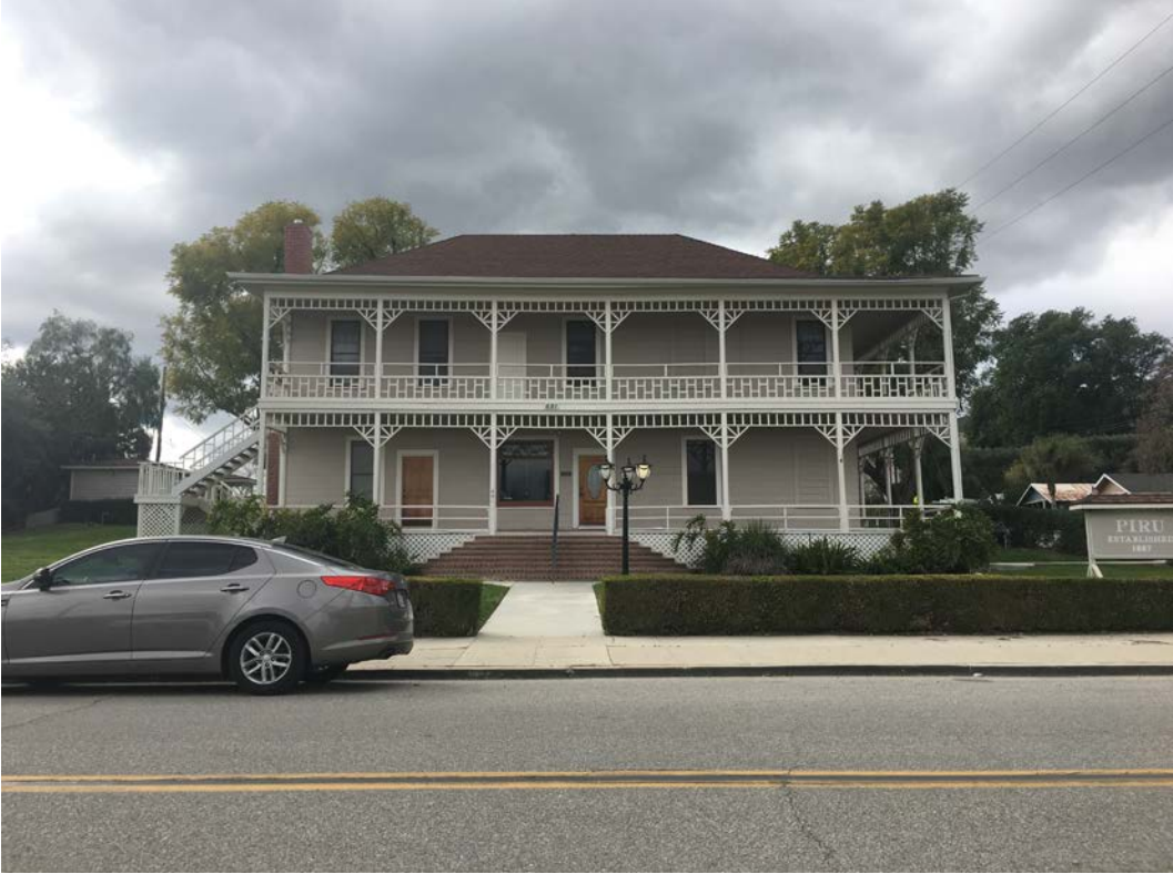
Front of Primary Structure (East Side)
