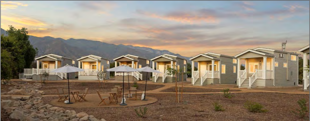
Photo of the constructed Mesa Farm Tiny Home Community; Photo credit: Upmarket Media
